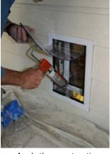
Apply the construction adhesive directly to the sides carpet inward and place and bottom of tunnel.
