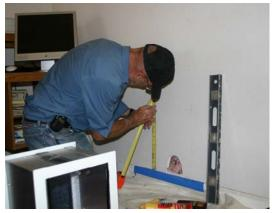
Measure and mark the hole carefully, making sure it is square and level.
