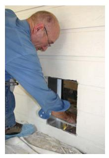
Step 17: Insert the inside frame and tunnel back into the opening. From the outside, pull the inside door frame tightly against the inside wall and push the flashing snug against the outside wall.
