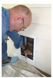
Sleeve outside frame into tunnel and pull firmly together.
