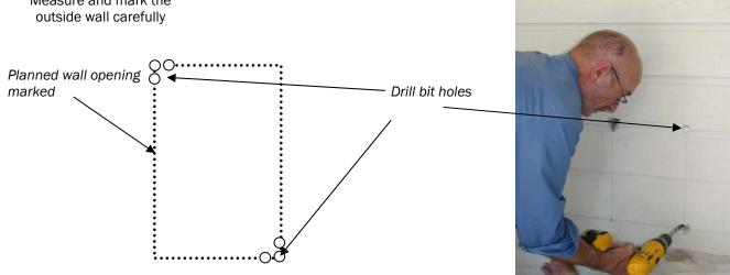
Drill out corners first to make it easy to insert saw blade.
