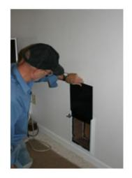
Installing the standard top loading security cover. It can also be ordered side-loading.
