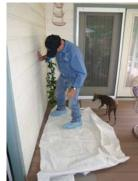
**Step 6:** Draw a pattern on the inside wall according to your pet door size with a pencil. Wall openings are listed below according to pet door size. For special size pet doors the opening may be determined by measuring the tunnel. Make sure your opening is square and level.
