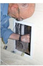
Carefully unroll the carpet pressing firmly against sides and bottom of tunnel.
