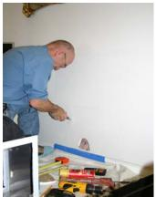
Cut the opening with a drywall saw.
