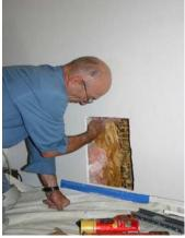
Push the insulation into the wall out of the way.
