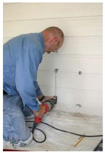
A reciprocating saw easily cuts the exterior hole, although other types of saw can be used.
