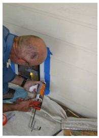
Tape and caulk around the door perimeter to seal the pet door. DO NOT caulk the outside.
