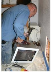
Use tin snips to cut the tunnel to the correct depth.
