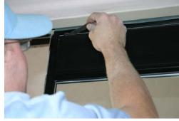
**Step 11:** Slide the stationary panel away from the Hale Omni Panel™ Insert so you can access the edge of the Hale Omni Panel™ Insert.
