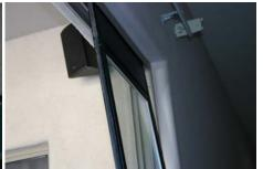
Step 9: With your hand, push the "U" channel (Figure 2 E) up securely into the top of the track (Figure 2 Door Channel). Pull the sliding plate (Figure 2 B) down to expose the adjusting nuts. (Figure 2 A)
