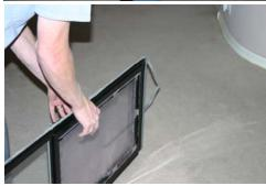
Unroll grey weather- stripping and feed into channels on both sides of the Hale Omni Panel™ Insert. If you use the Omni extension, leave the weather-stripping off that side.
