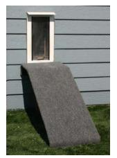
**Step 3:** If possible, make sure the installation location has a fairly level surface. If you are installing your ramp in an exterior location, you do not want the ramp to "rock" on uneven ground.
