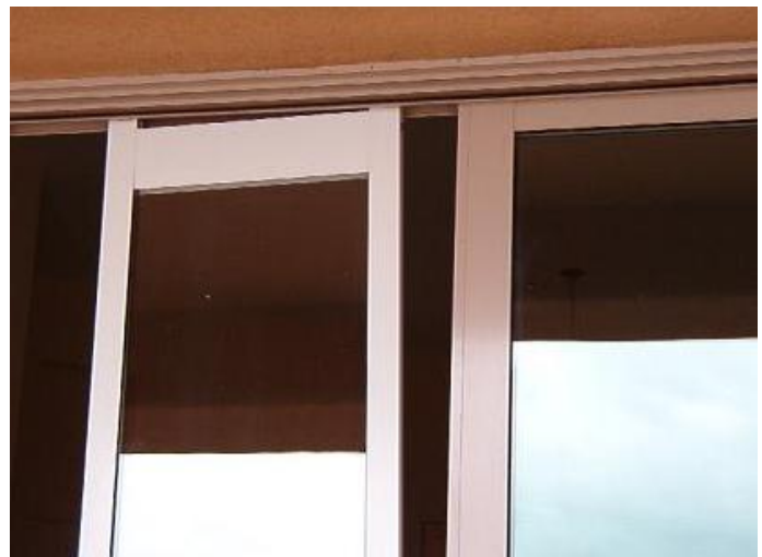
Test fit the panel insert into place.
