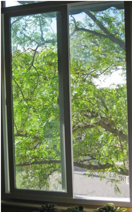
Sliding window with original screen panel in place.
